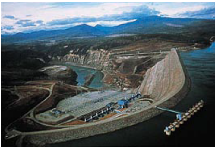
The WAC Bennett Dam holds back the largest reservoir in North America.
